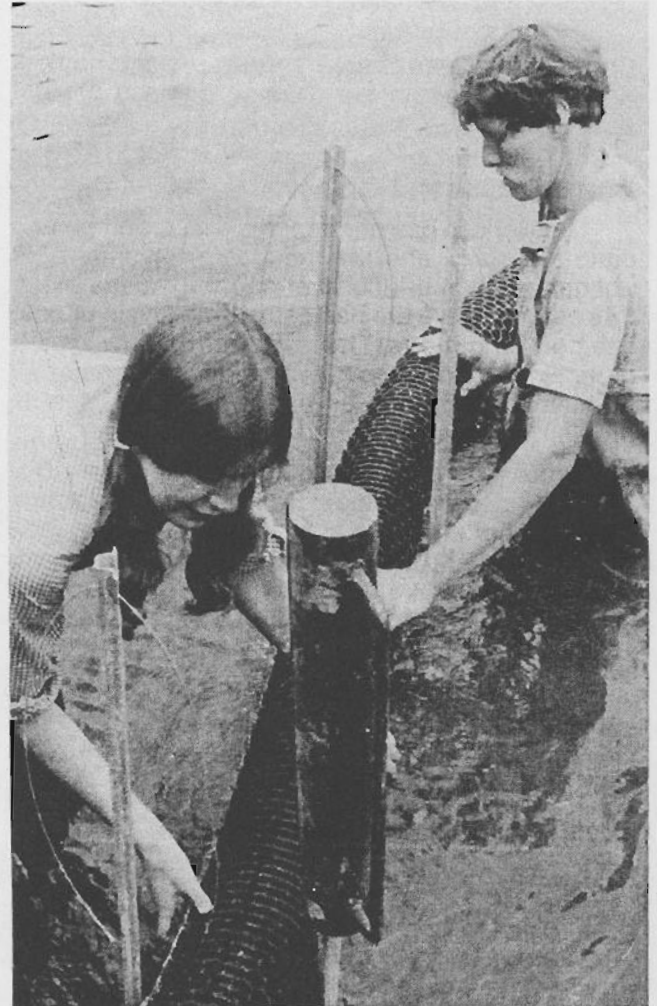
When the pipe is put in place, it should be secured by stakes or posts.
